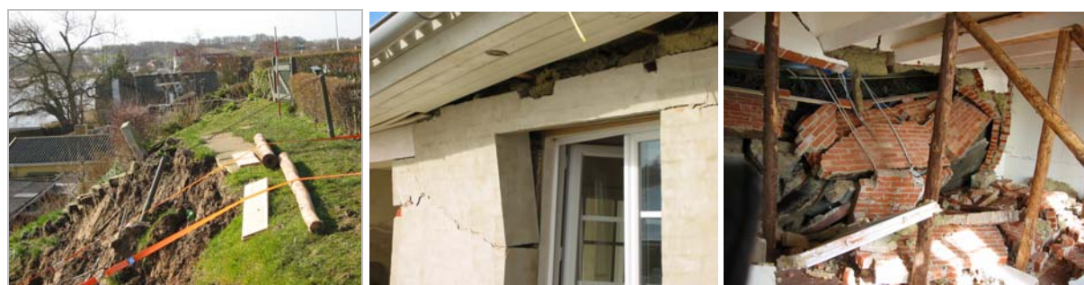
Figure 1. Dire reality of a minor slope failure leading to total demolition of a one-family house in Denmark
