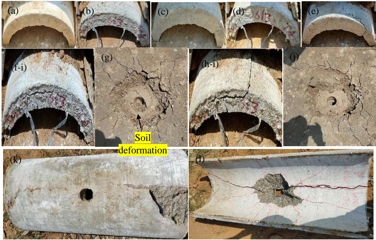
Fig. 9. Damage to tunnel side face (a-e) 1 st impact to 5 th impact, (f-i) 6 th impact, (g) damage to soil cushion layer for 6 th impact, (h-i) damage to side face for 7 th impact (j) damage to damage to soil cushion layer for 7 th impact and (k) & (l) front and rear face damage on 8 th impact
