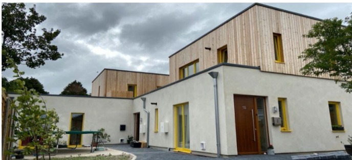
Image 4: The outside of one of the completed properties
