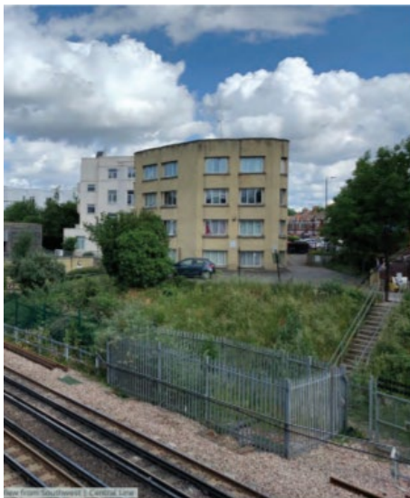
Image 2: The building before demolition
