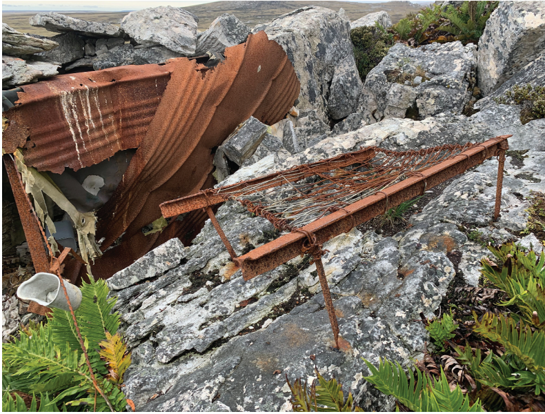
Figure 16. Probable seat base with sides from angle iron and sprung support provided by wire mesh. Shelter and wall of oil drum sheeting in background.
