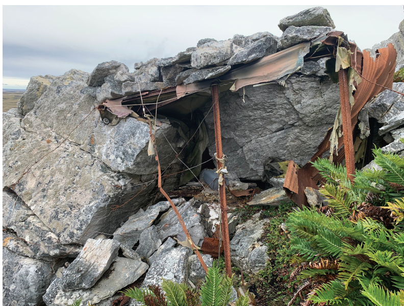
Figure 15. Possible observation post shelter. Note rocks on roof and sheeting from recycled barrel forming wall to right behind heavy girder upright in corner.
