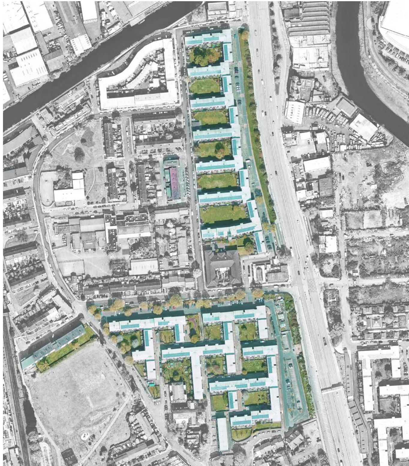
Aerial view of the Teviot Estate
