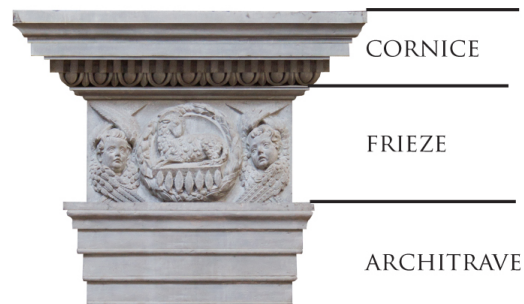
CORINTHIAN ENTABLATURE OF THE COLUMNS IN THE NAVE OF THE BASILICA OF SAN LORENZO (1450 ET SEQ.)
