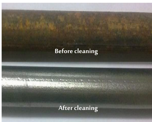
Fig. 2. The steel bar before and after the cleaning phase
