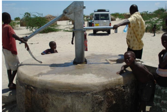
Figure 2. The current water supply in Longech village: an Afridev pump (picture kindly supplied by Brian McSorley)
