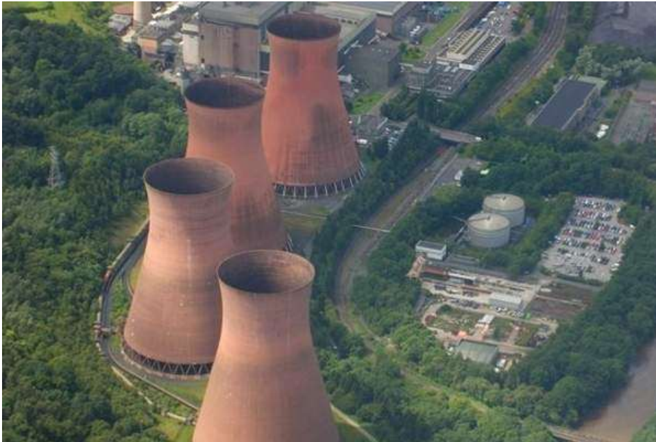
Figure 2-16 The Ironbridge power plant at Severn Gorge, UK (Power stations of the UK, 2019)
