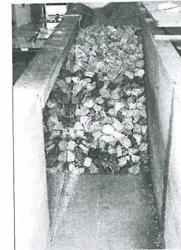
Armour layer placed
