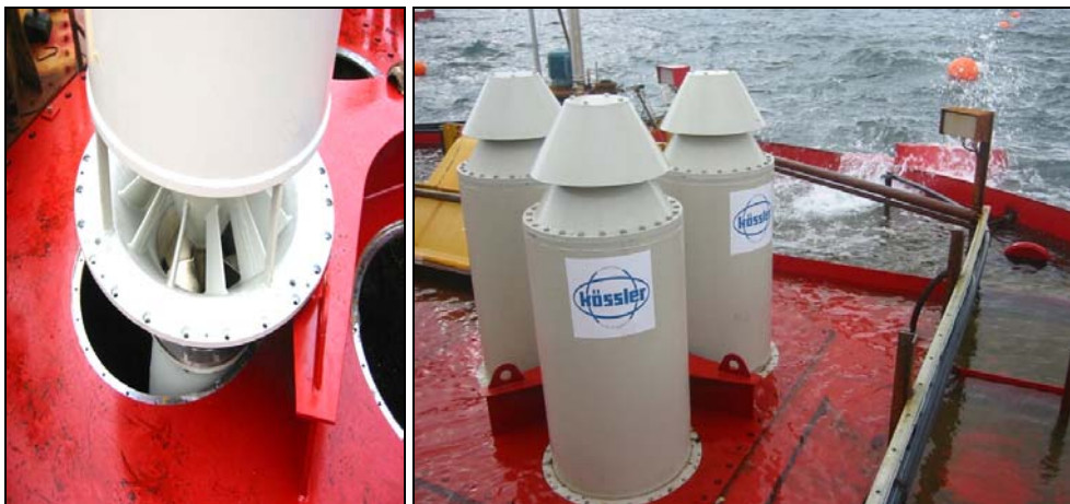
Fig. 4.13 Installation of draft tube and installed turbines.
