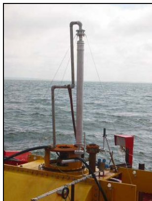
Fig. 4.2 Large diameter pipe installed in aeration tube
