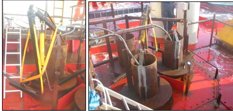
Fig. 4.6 Hoist used for dummy turbine removal and dummy turbines following maintenance
