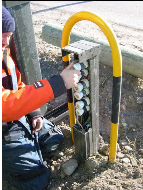
Fig. 2.1 Connection of WD to the grid
