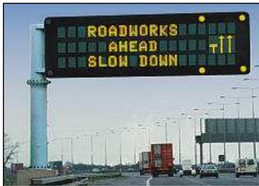
Figure 6: MS3 signs are being rolled out on the UK Motorway Network as part of the National Traffic Control Centre Project (source: The Highways Agency)
