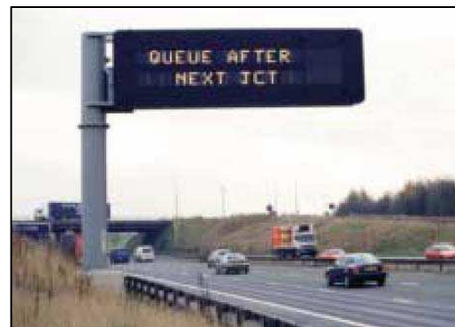
Figure 2: Tactical VMS notifying motorist of queue ahead (source: The Highways Agency)
