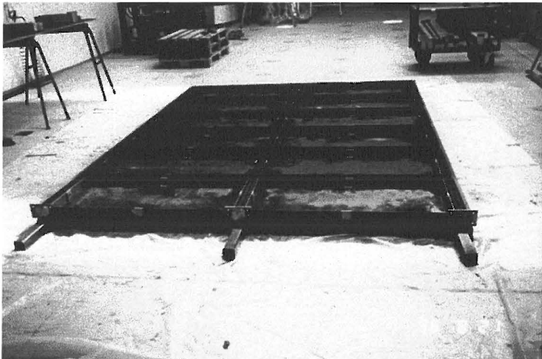
Figure A.1: The form used for construction of the frames.
