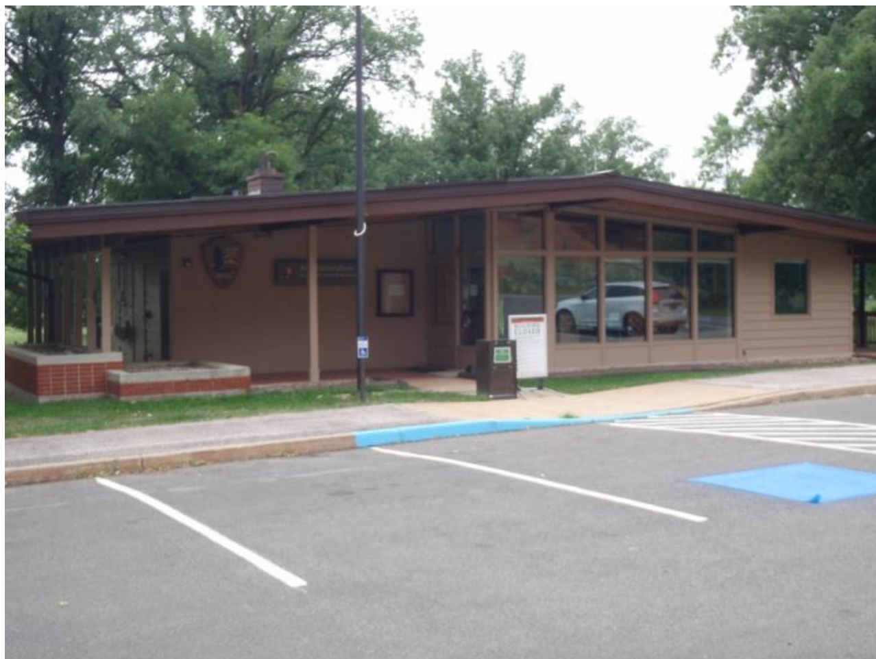
Figure 28. Mission 66 Administration Building in the area by the Belle Fourche River. The modern stylistic elements of the Mission 66 era appear in this structure's one-story, the large, low-pitched front gable roof, accents of brickwork, and a façade curtain wall. (Photo by Janet Ore, June 2020).
