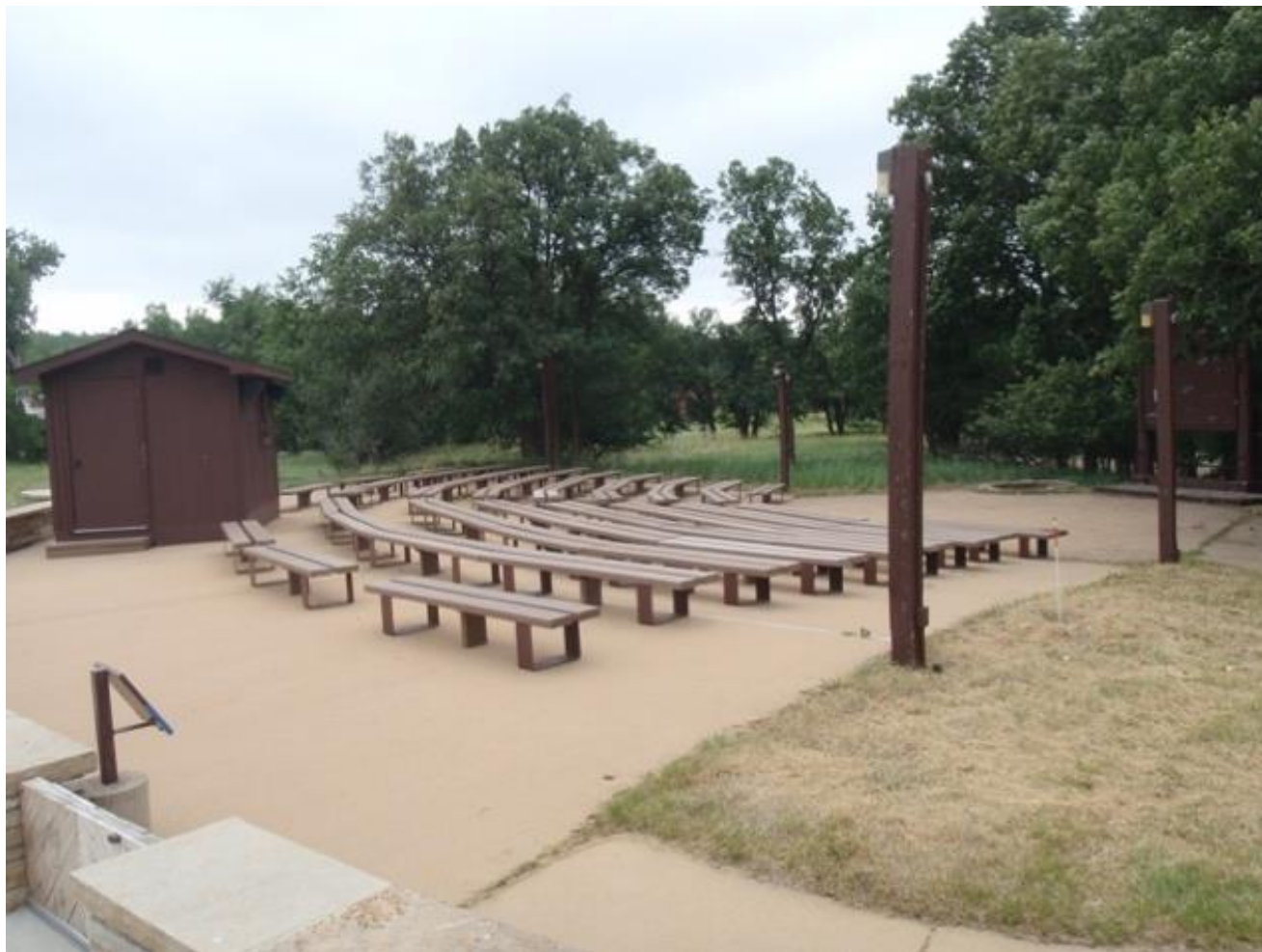
Figure 30. Amphitheater constructed during Mission 66. The seating capacity was expanded, and a structure to house audio-visual (AV) equipment was added. The fire pit previously existed as a focal point. (Photo by Janet Ore, June 2020).
