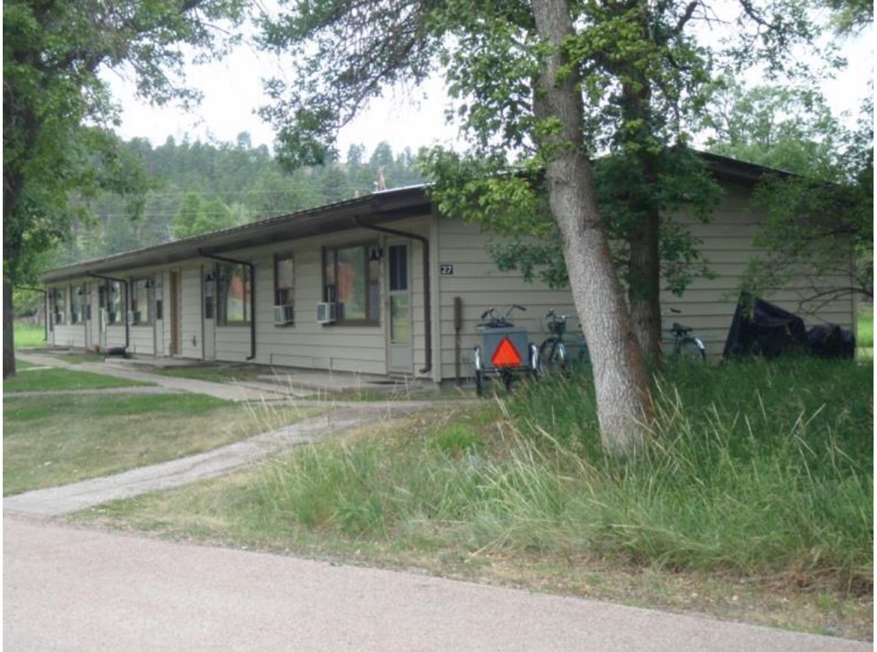
Figure 29. Mission 66 Employee Housing. In this building, a multi-unit apartment with shared utility and storage spaces. (Photo by Janet Ore, June 2020).
