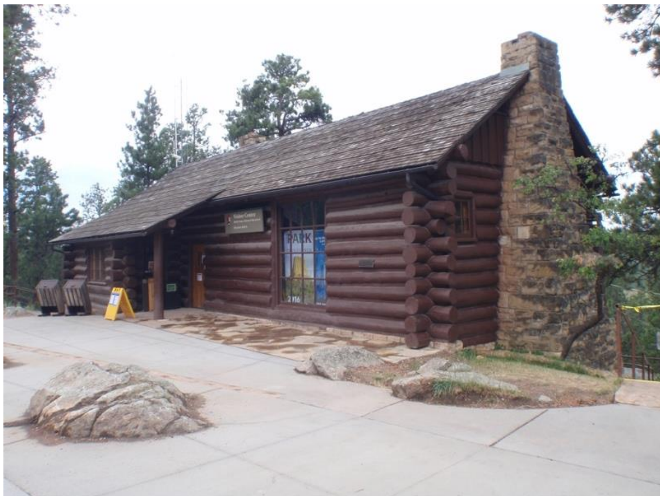
Figure 25. Visitor Center. (Photo by Janet Ore, June 2020).
