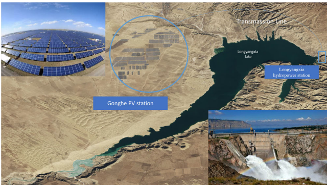
FIGURE 7 Layout of Longyangxia hydro-PV plant.
