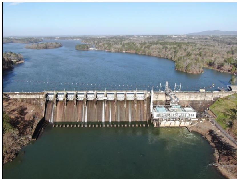
Figure 3.5: Photo of the Carpenter Dam located near Hot Springs, Arkansas (Image from Entergy Arkansas, LLC.).
