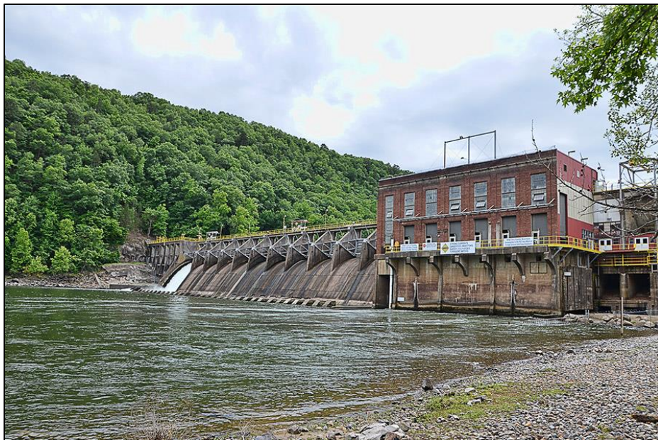
Figure 3.4: Photo of the Rempel Dam located at Magnet Township, Arkansas (Image from the Arkansas Historic Preservation Program).
