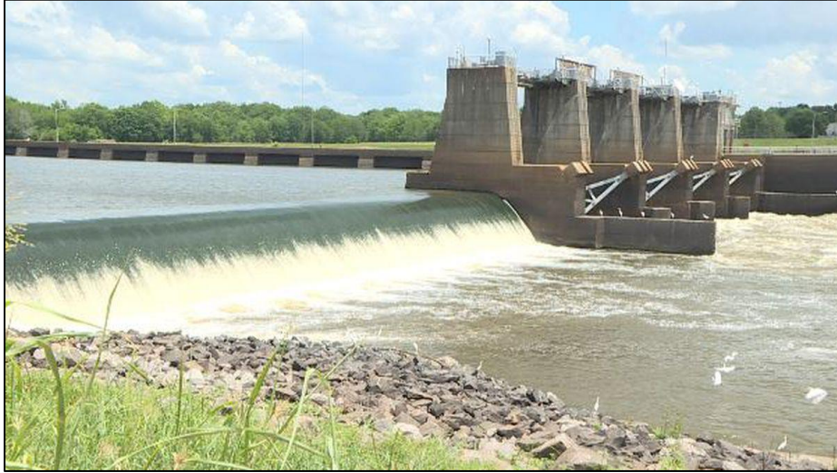
Figure 3.3: Photo of Columbia Lock and Dam located in Columbia, Louisiana (Image from KNOE 8 News).
