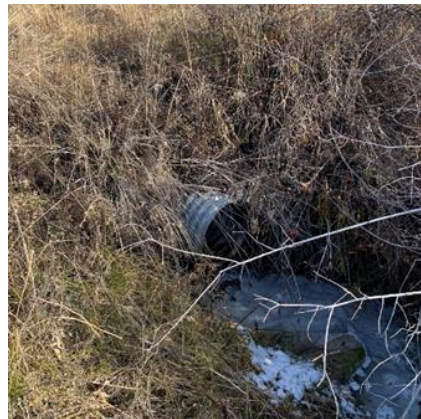
Figure 32. Photo of culvert on the Porcupine Creek.
