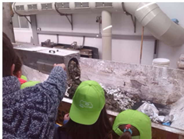
Figure 1. Educational visit to wastewater pumping station. Source: own elaboration.
