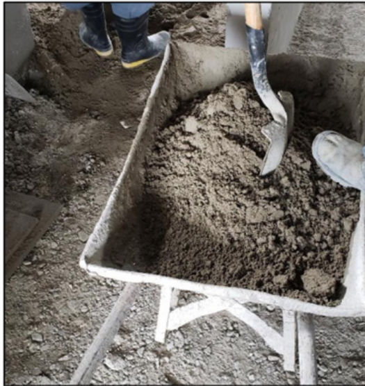
Figure 12: Transporting the mortar.
