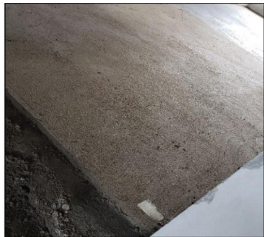
Figure 15: Final result of screed.
