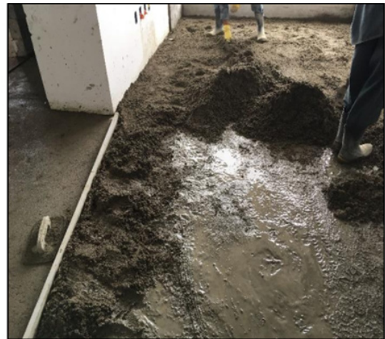
Figure 14: Base sprinkled with cement.
