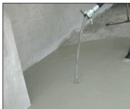
Figure 7: Launching SLS on the surface [11].
