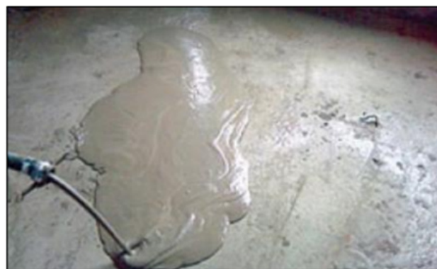
Figure 6: Fluidity of the self-leveling mortar [14].
