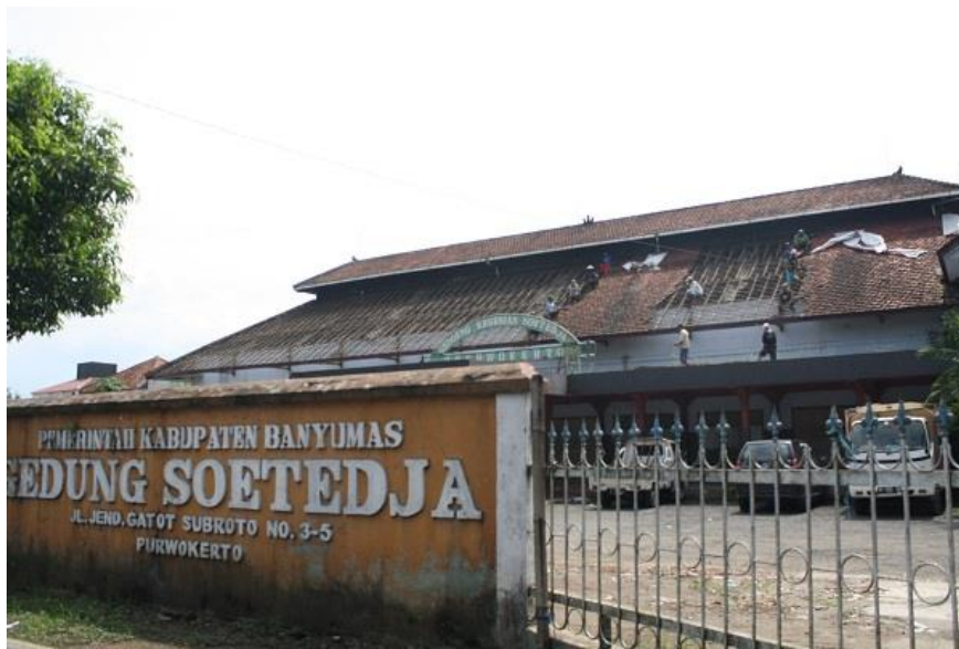
Figure 5. Demolition of Gedung Soetedja on 2015 (Source: NPS documentation)
