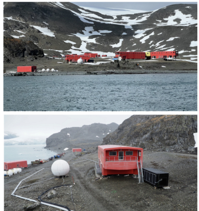
Fig. 1. Upper picture: a general view of BAE-JCI. Down picture: MazORCA (the ORCA's black container) close to the scientific module building (red building) and the communication antenna (white igloo).
