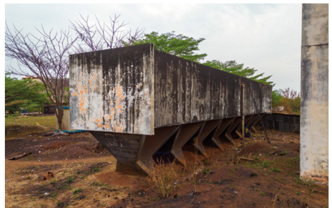
02 The water tower and tank, University of Nigeria Nsukka (Enugu Campus), Enugu, Nigeria. © Ikedi Chukwuka, 2023.
