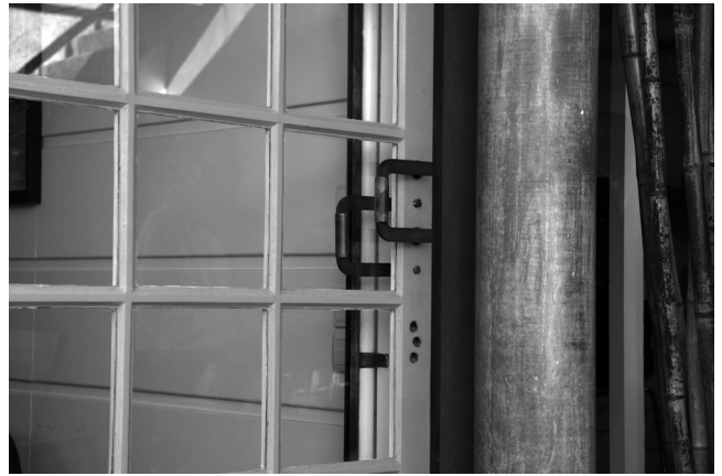
05 Álvaro Siza, Manuel Magalhães House, Porto, Portugal, 1967-1970. Window detail. © Ana Tostões, 2020.
