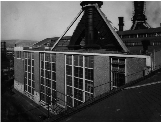
04 Virgil Bierbauer, Kelenföld Power Plant, Budapest, Hungary, 1925–1934. Boiler house III, 1931–1932. © Hungarian Museum of Architecture and Monument Protection Documentation Center – HMA, Tivadar Kozelka, 1934.
