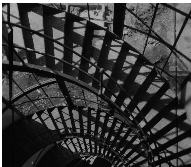
07 Virgil Bierbauer, Kelenföld Power Plant, Budapest, Hungary, 1925-1934. The stairs of the switch-house under construction as it was photographed by Virgil Bierbauer. © Hungarian Museum of Architecture and Monument Protection Documentation Center - HMA, Virgil Bierbauer, ca. 1933.
