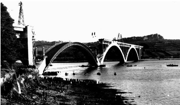
Figure 13. The bridge being rebuilt.
