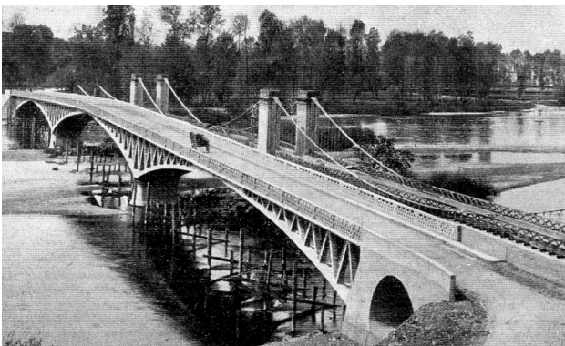
Figure 7. The Veurdre Bridge immediately after its construction.
