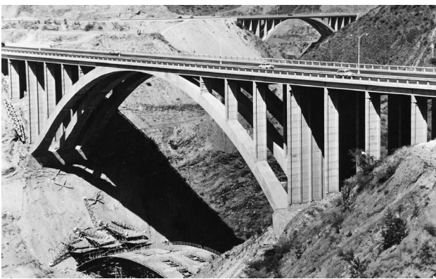
Figure 29. Two of the bridges with a 150-metre-long span upon finishing the highway.
