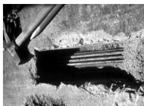
Figure 4. The prestressed bars
