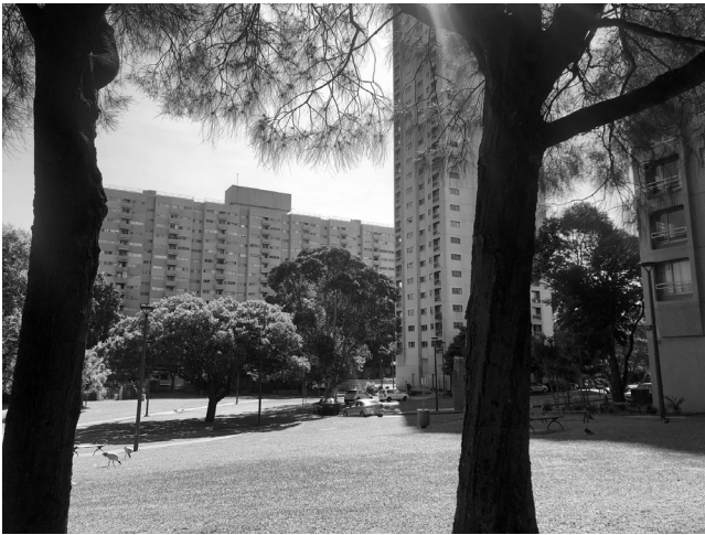
05 Stafford Moor and Farrington, Endeavour Project housing, Waterloo, Australia, 1976. Current view. © Noni Boyd.
