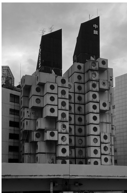
01 Kisho Kurokawa, Nakagin Capsule Tower Building, Tokyo, Japan, 1972. Full view of the Nakagin Capsule Tower. © Tatsuyuki Maeda, 2020.
