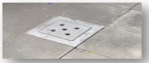
Gambar 6. Lubang resapan biopori
