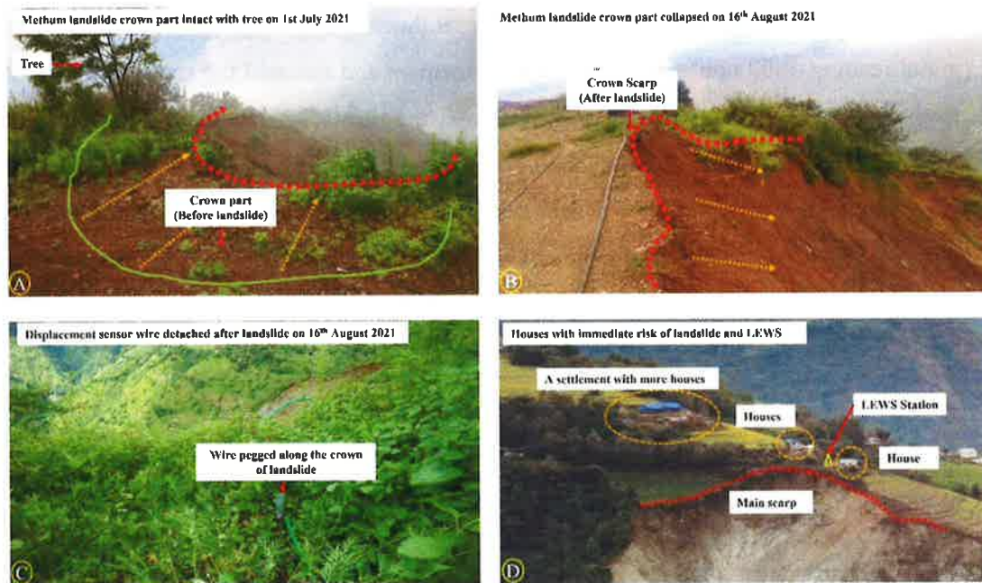
Figure 10. Methum landslide crown failure and vulnerable households: (A) head scarp of the Methum landslide as of July 1, 2021; (B) the scarp following the collapse on August 16, 2021; (C) detached wire from the displacement sensor on August 16, 2021; (D) houses and settlement above the landslide's main scarp.
