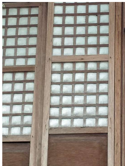
Figure 1. Example of a traditional Capiz window (photograph JMR, 20 June 2023, Samal, Bataan, Region III, Philippines).
