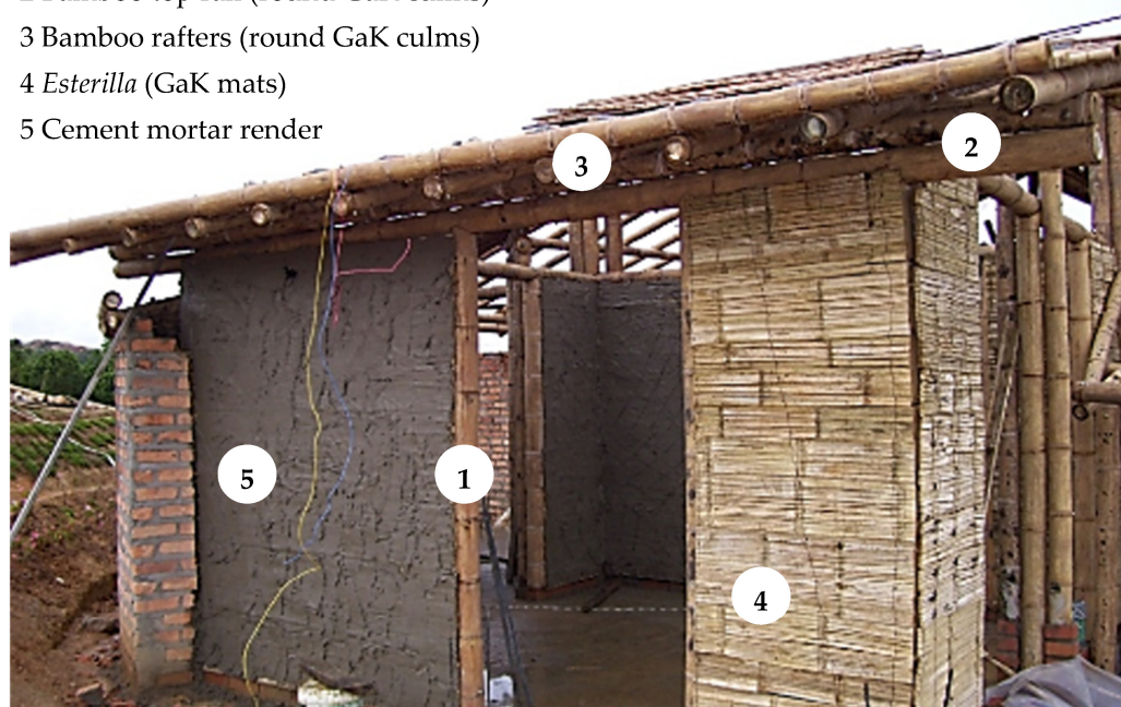
Figure 2. Light cement bamboo frame (LCBF) system.
