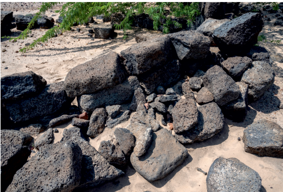
Fig. 7: Detail of the constructive technique of a house wall, where the inner rubble infilling can be appreciated.
