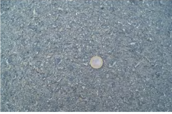
Fig. 2. Detail of the road surface on which tests were conducted.
