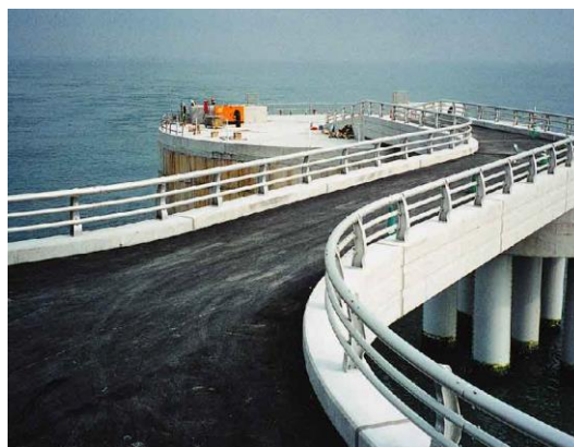
Figure 2.4.3 Haramachi Thermal Power Plant Outfall Bridge
