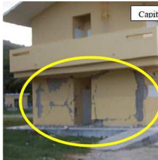
Figure 2. Illustration 40, web crushing. Source: Moreno (2014)
