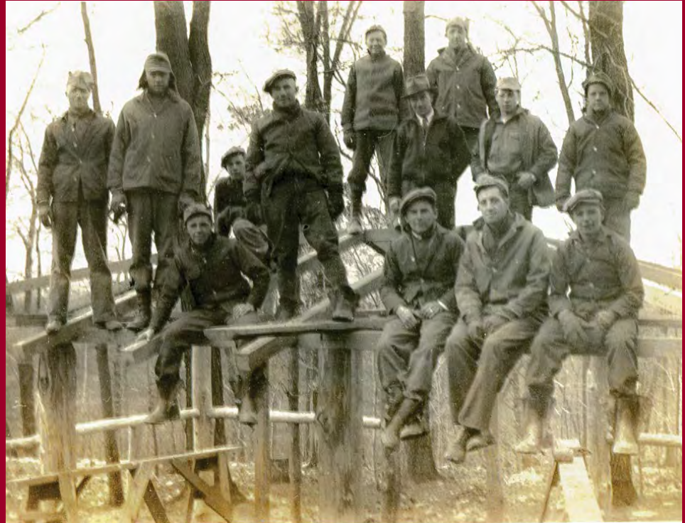
One of the many early projects assigned to work crews was the construction of large barracks buildings at the camp site.
