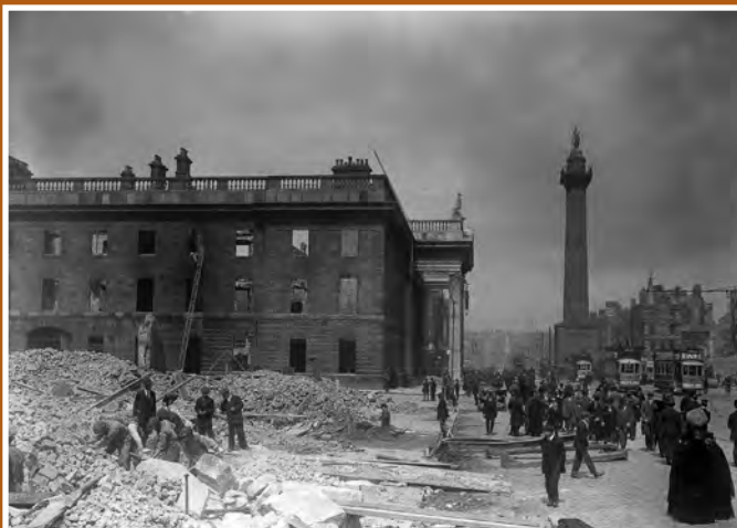
The shell of the G.P.O. on Sackville Street (later O'Connell Street), Dublin in the aftermath of the 1916 Rising. Date: May 1916
