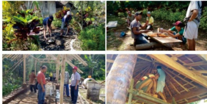
Figure 2: Cooperation activities to build facilities at KBG
