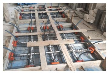
Figure 3: Details of reinforcement steel.
