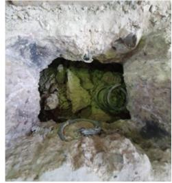
Figure 7: A picture to illustrate the shape of the opening after casting, as well as the cut strand after tension.
