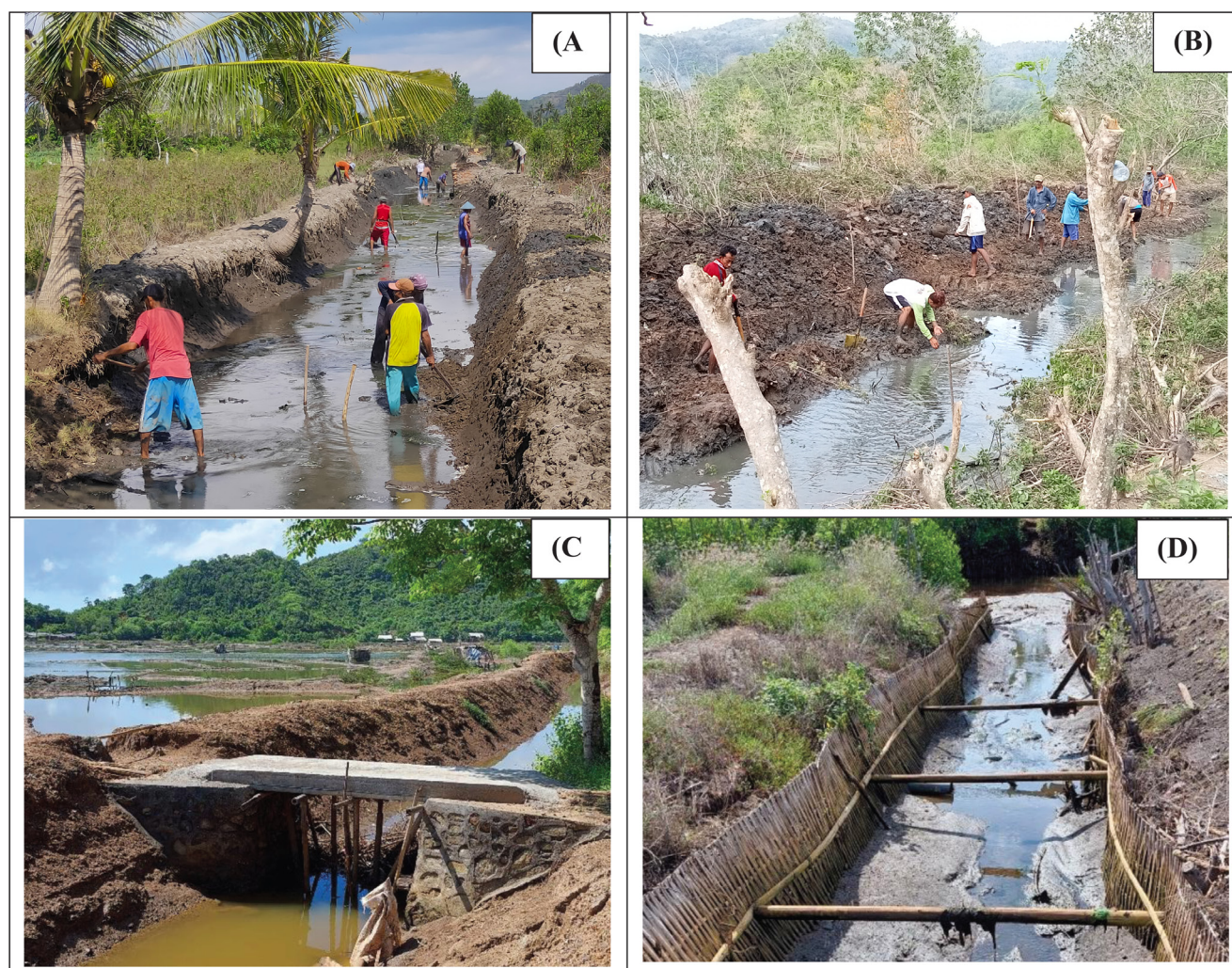
Figure 2 Images of collective action to maintain the irrigation canals in: (A) Lembar in 2022 and (B) Sekotong in 2022. Images of (C) Jerowaru and (D) Sambelia, were taken in 2021 after collective maintenance was completed. All photos were taken by first author during fieldwork in 2022.
