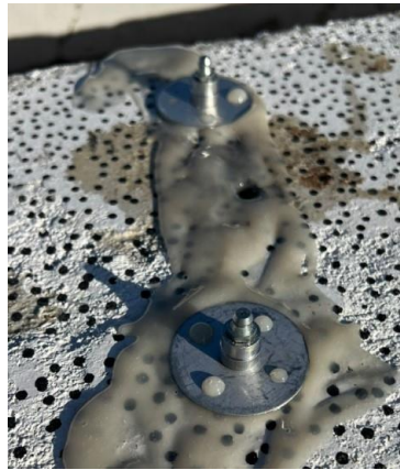
Figure 9. Surface packers secured with nails
