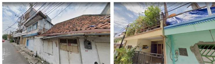
Figure 3.7 . Modern building typology Google street view, 2023
