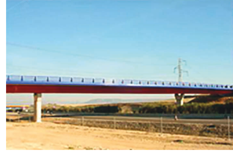
FIGURE 1: The Magaz bridge.
