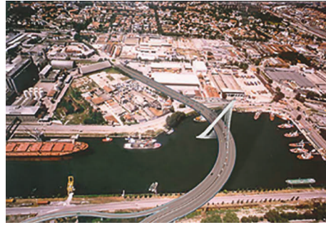
FIGURE 7: The curved cable-stayed bridge of the Porto Marghera (Venice, Italy).
