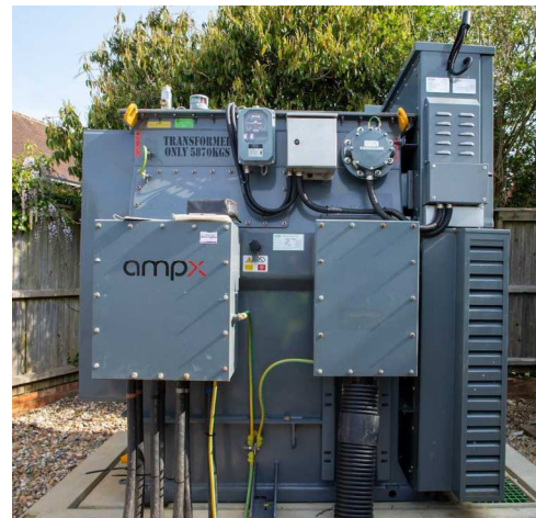
Figure 8: Amp X Smart Transformer on the distribution network in the UK.
