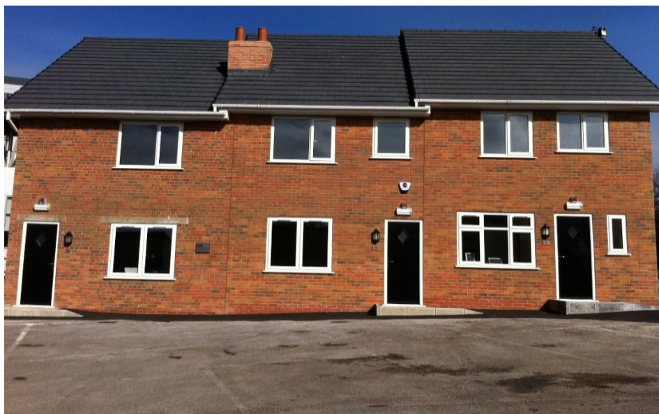
Figure 1. LJMU's exemplar houses, which include three houses that are constructed to emulate domestic houses from different eras (1920s, 1970s and 2010s).
