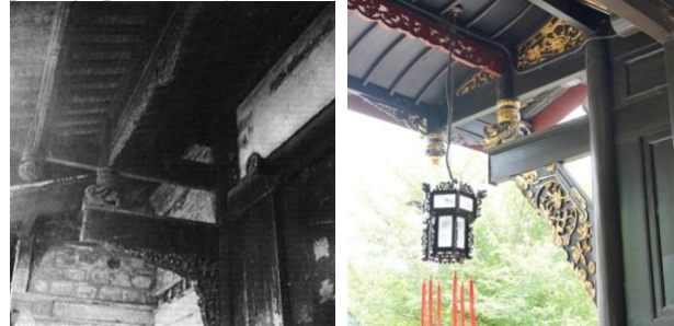
Figure 3. The difference in tectonic under the eave of the Chen House: before and after the restoration, left © Z. Liu 2000, right © the author 2019.
