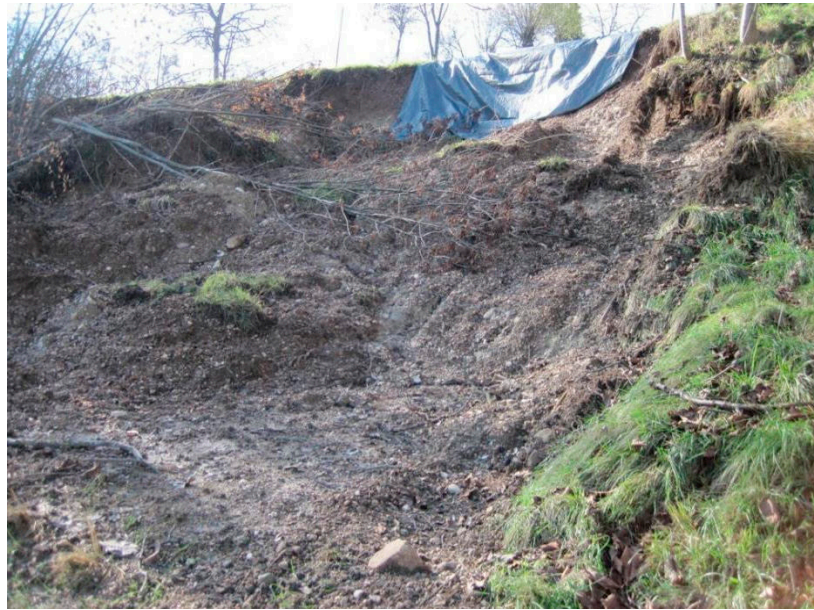
Figure 9. Landslide photograph code 025021_06c.
