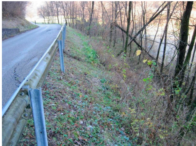
Figure 10. Landslide photograph code 025021_07c.
