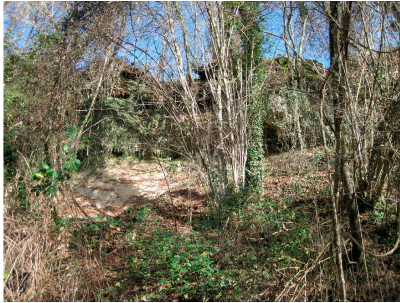
Figure 7. Landslide photograph code 025021_05c, rotational sliding.
