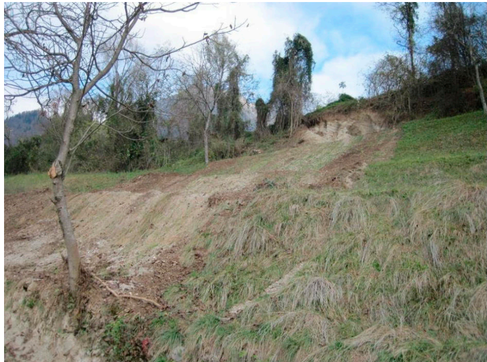
Figure 4. Landslide photograph code 025021_02c.
