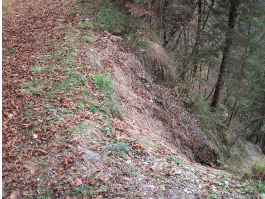
Figure 5. Landslide photograph code 025021_03c.
