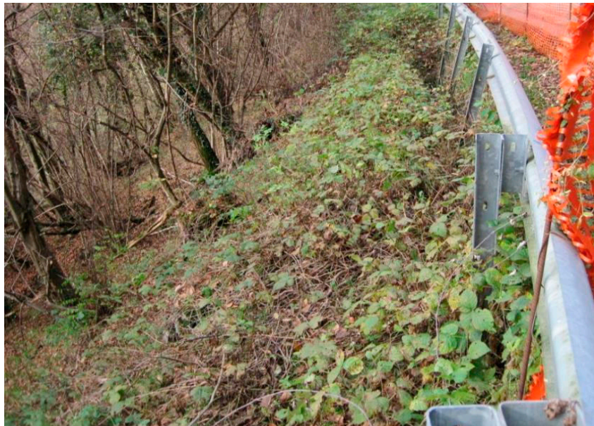
Figure 6. Landslide photograph code 025021_04c.
