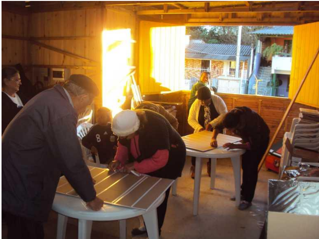
Figure 10 – Applying double-sided adhesive tape in cardboard sheets – Source: The authors
