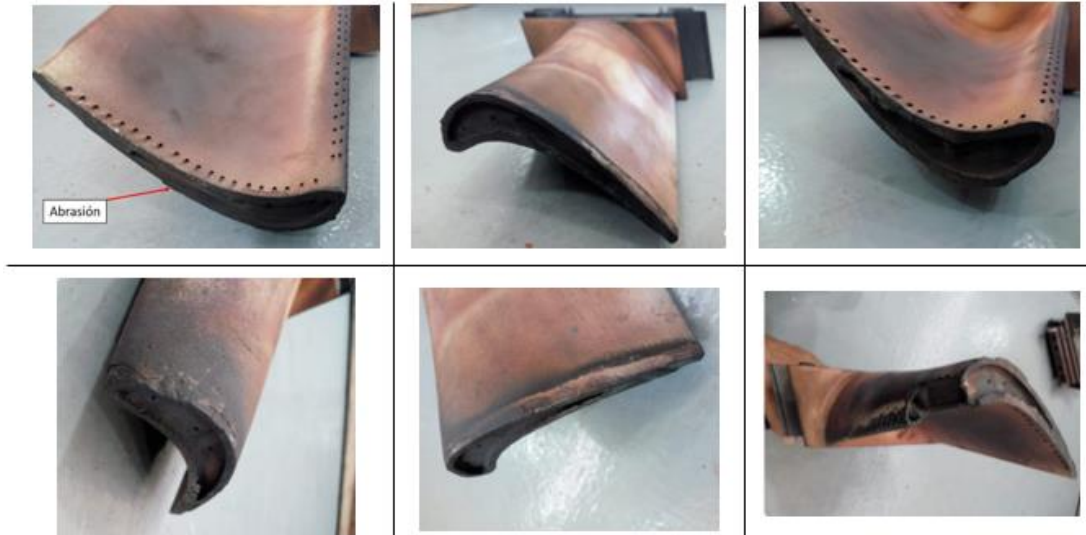
Figure 2. Some typical defects in degraded blades
