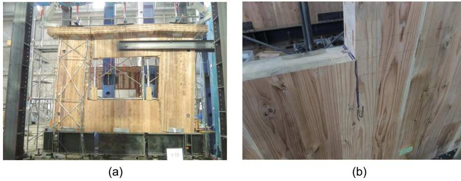
Fig. 1. Corner cracks with CLT panels with openings: (a) in-plane load testing; and (b) details of the cracked section.
